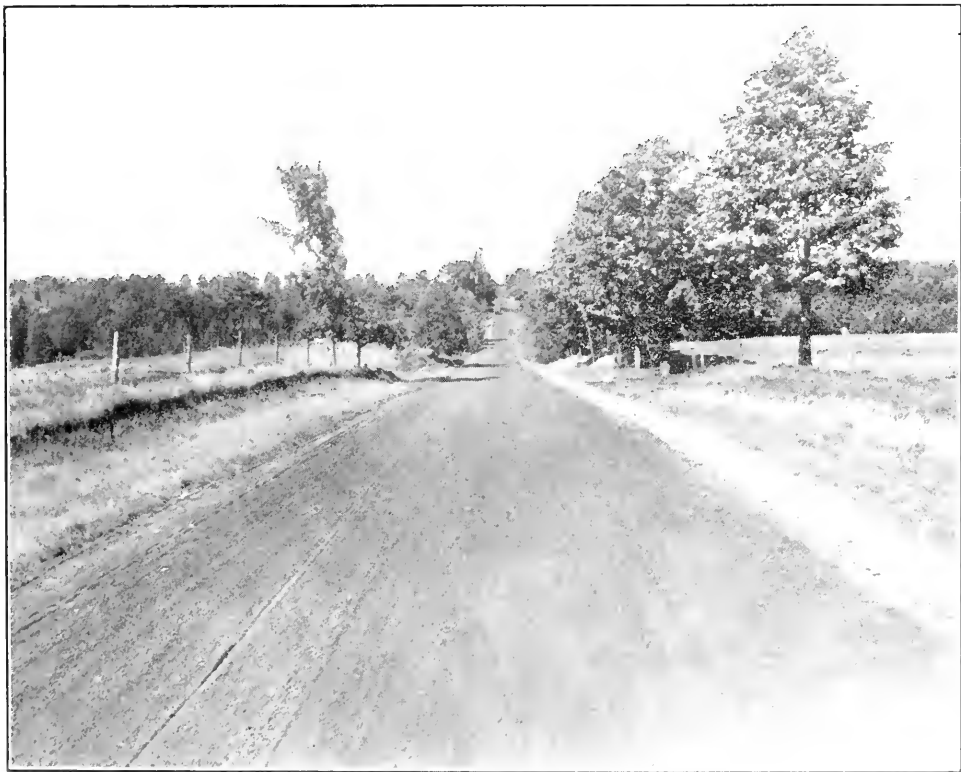
Gravel road maintained by ordinary dragging. Treated with \frac{1}{4} -gal. gravel dust-laying oil. Langstaff-Brooklin Highway.
